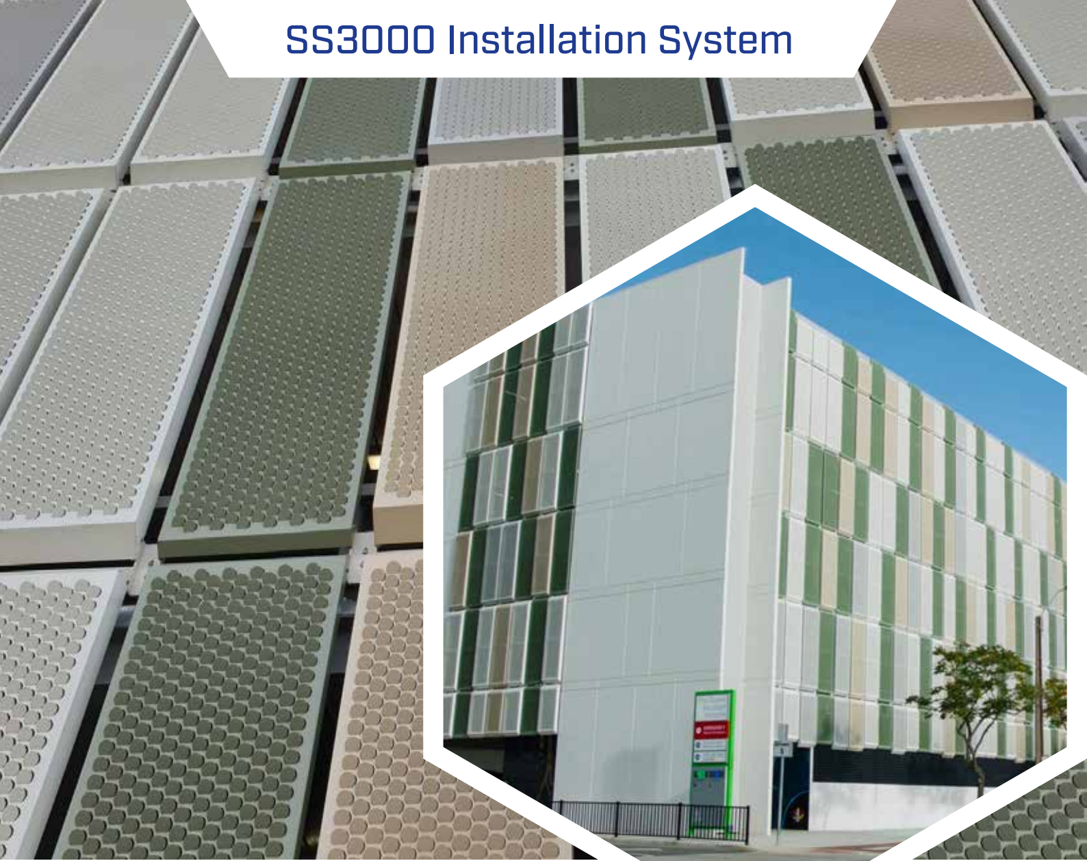
The Queen Elizabeth Hospital Carpark SA
